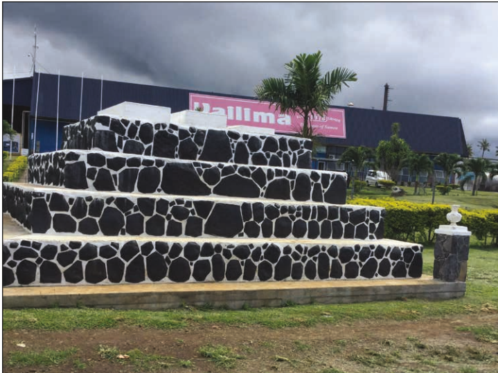
Figure 4. Mataia tia at Vaitele after renovation.
