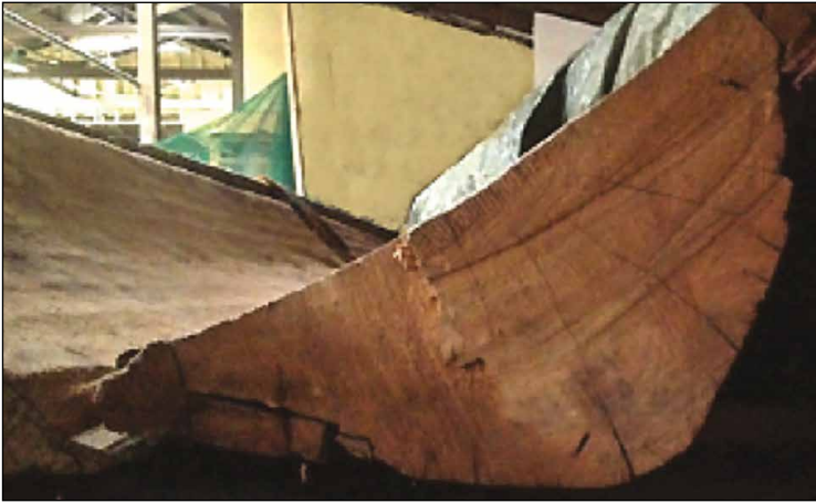
Figure 5. Curved under-surface of the tāhuhu of Whare Mataatua, Whakatane. Photo by J. Treadwell (2013); used with permission of Ngāti Awa.
