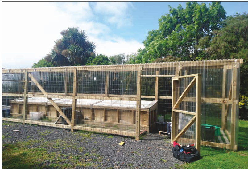
Figure 17. Purpose-built satellite conservation facility at Ōtākou Marae, Otago Peninsula. The polycarbonate-clad enclosure provides dry, secure storage for conservation chemicals and promotes higher temperatures during cooler months of the year to facilitate treatment progress. Additional shelving and small tanks have now been installed to accommodate the continuous stream of artefacts as they are recovered.
