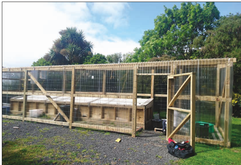
Figure 17. Purpose-built satellite conservation facility at Ōtākou Marae, Otago Peninsula. The polycarbonate-clad enclosure provides dry, secure storage for conservation chemicals and promotes higher temperatures during cooler months of the year to facilitate treatment progress. Additional shelving and small tanks have now been installed to accommodate the continuous stream of artefacts as they are recovered.
