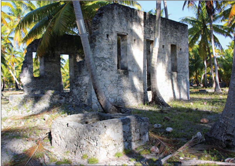
Figure 3. Early historic house and well, both made of coral blocks, in Hökikakika. Author's photo, 2019.
